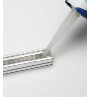
6. Apply silicone along sides where the lens will rest. Make sure to leave a small section on one side without silicone to allow air to escape while installing lens.
