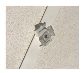
Install the clip in the T-Grid by pressing, then secure by twist until it is adjusted.
