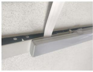
Carefully bend the flat wire at the edge of the T-Grid, giving it the same shape of it.
