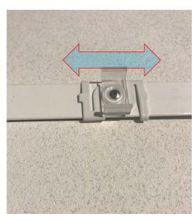
Once Clip is installed slide trough the T-Grid until it is located in the right position.
