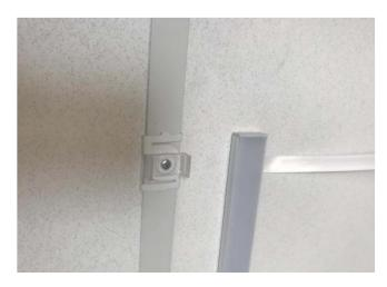
Carefully press the fixture inside the brackets, the leap in the plastic bracket will secure the fixture in the channel of the aluminum profile
