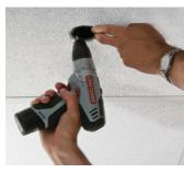
Insert fixture through  $2\,\%$ " cutout in ceiling,  $2\,\%$ " is standard hole saw size. Hinged design requires only  $5\,\%$ " plenum depth (Non-IC).
