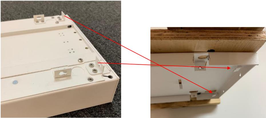
5. Lock in the other end and secure 4 corners – two on the ends and one on each side.
